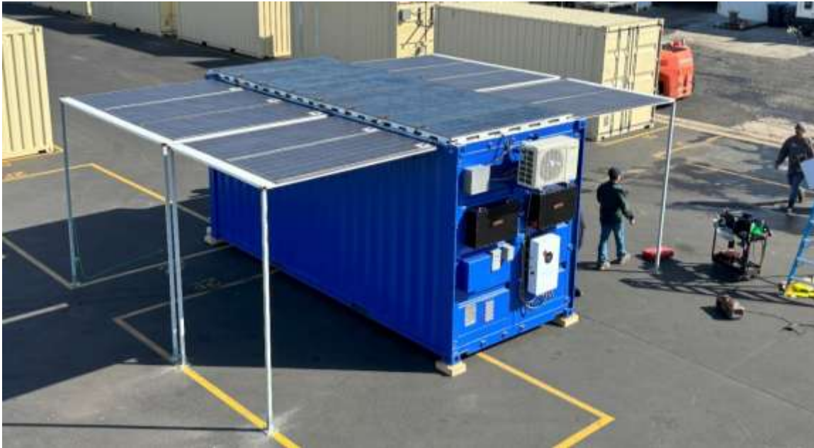
Figure 6.9. Containerized solar power system. Merlin Solar panels integrated onto a relocatable container provide immediate, fuel-free electricity for a pop-up energy system.
